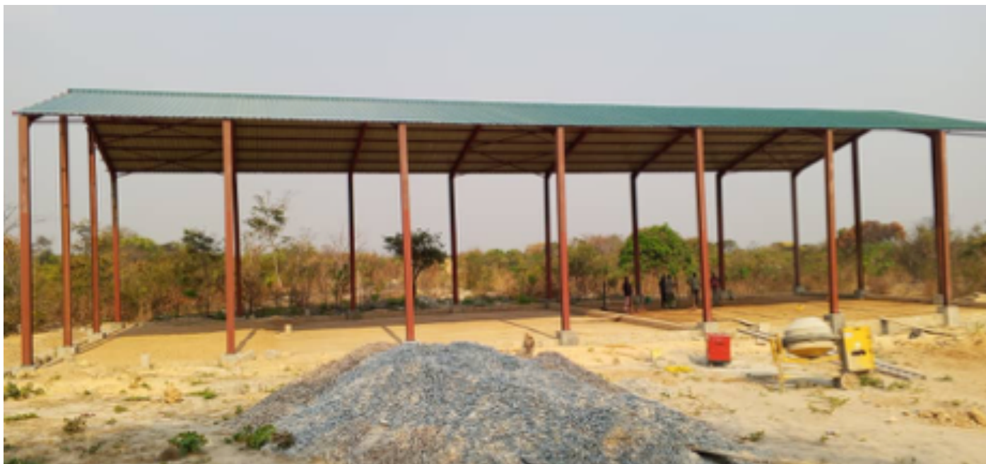
Figure 1 CEEC supported milling plant under construction in Chavuma.
