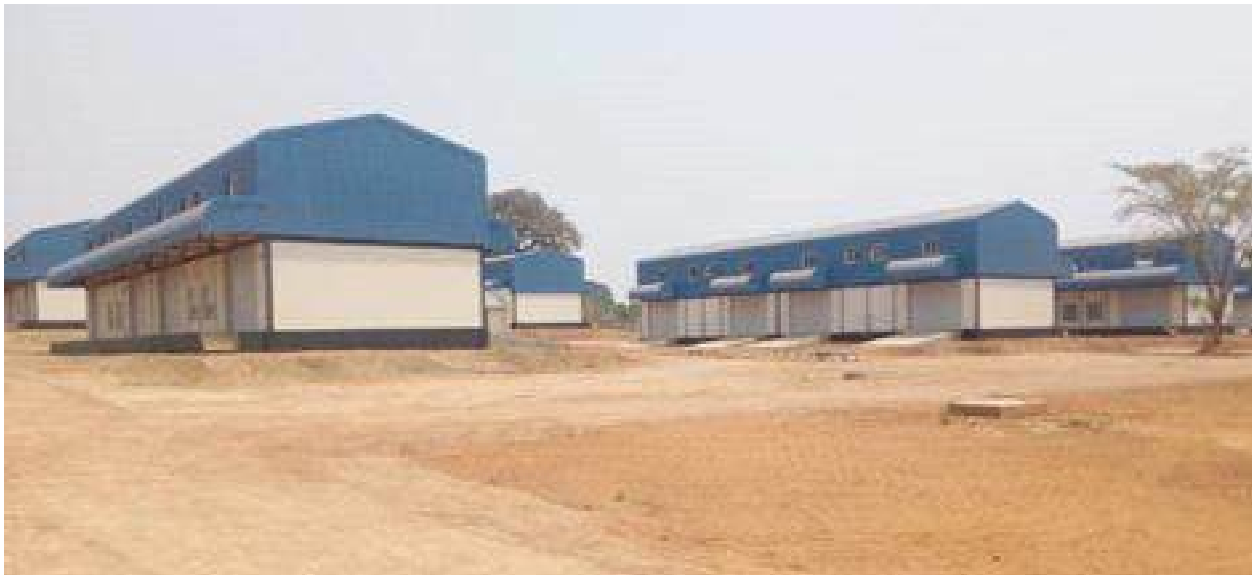
Figure 11 Kitwe Industrial Yard-General Workshops
