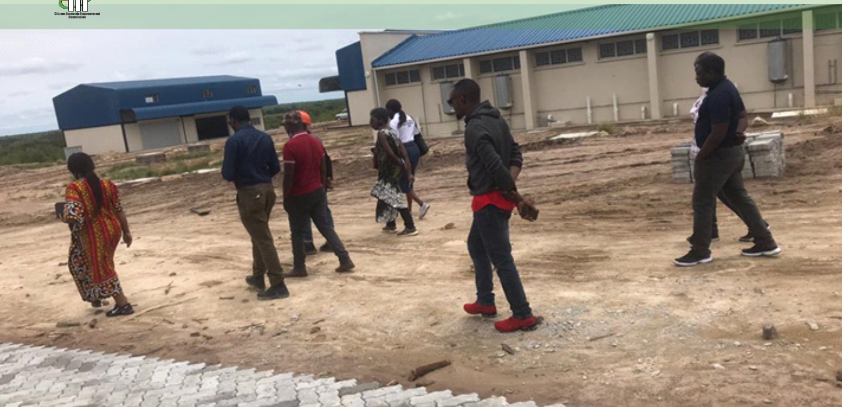
Figure 5 Commissioners touring the Mongu Industrial Yard.
