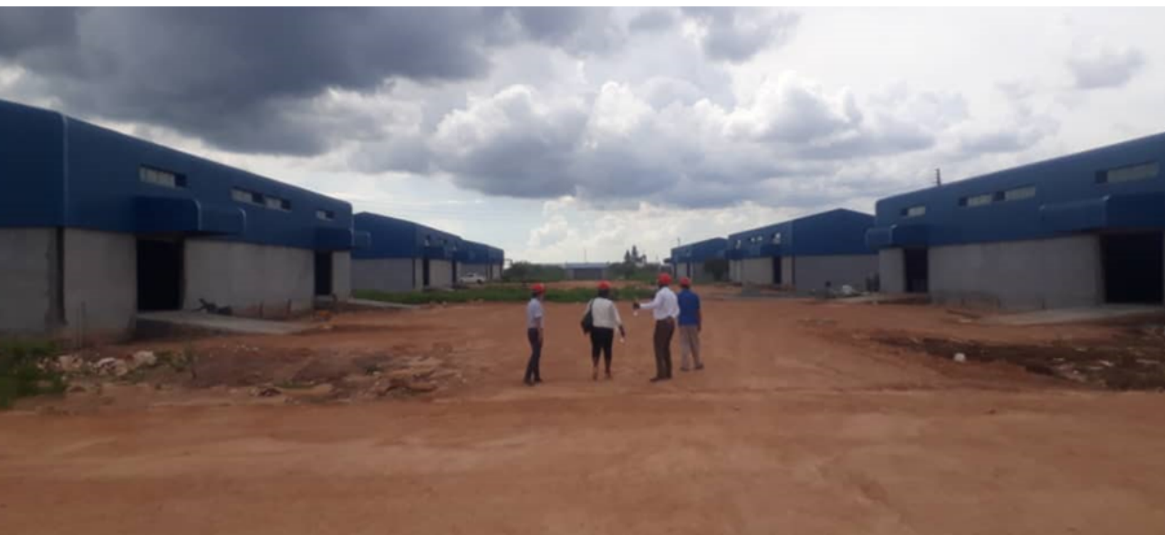
Figure 8 Lusaka Industrial Yard-General Workshops
